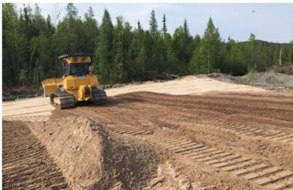
*Construction of the sand cover to shield radiation at Cayzor*
