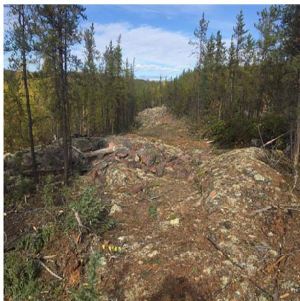
Tree clearing at Rix Smitty in preparation of remediation perimeter fence
