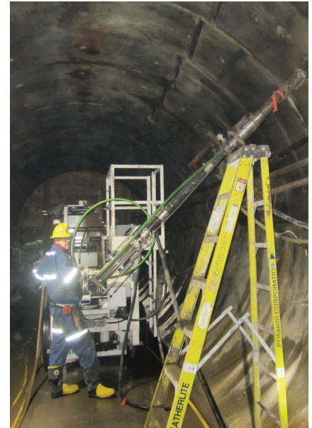
MBSS during surveying. Gamma probe and inertial probe were used to map this borehole. Probes were loaded into a borehole from an elevated platform located on the MBSS.
