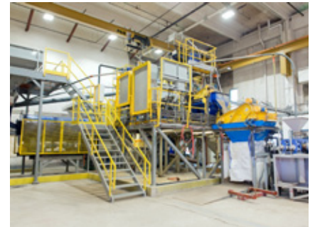
Completion: Physical installation of Kimberlite Ore Processing Facility.
