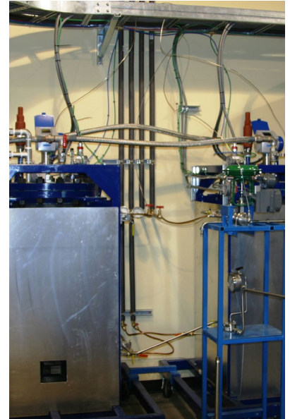
Production vessels and flow control valve.
