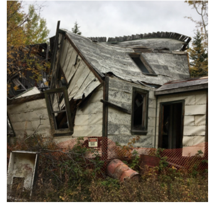
Photo 1: Nicholson - historical building to be inspected and demolished.
