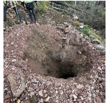
Photo 2: Murmac - mine opening to be covered with stainless steel closure.
