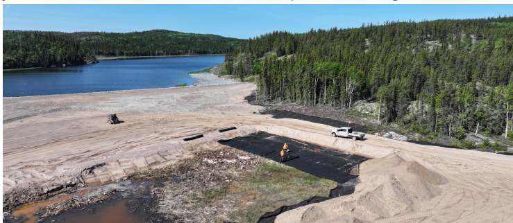
Photo 1: Drone footage of Langley Bay Tailings in 2025.
