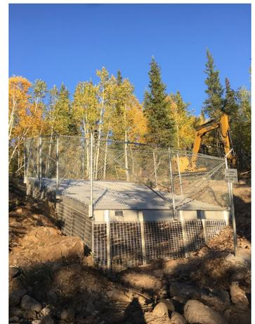
*Bat-friendly stainless-steel cover installed at Meta Uranium Mines, Beaverlodge Lake and Umisk Island. The closure is designed to allow bats in and out of the mine, as the opening provides a habitat for endangered bats.*
