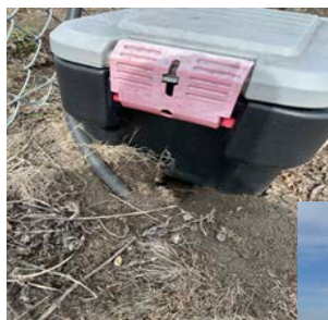
Some of the required infrastructure to operate a climate reference station April 30 2024 Photo: R. Jansen
