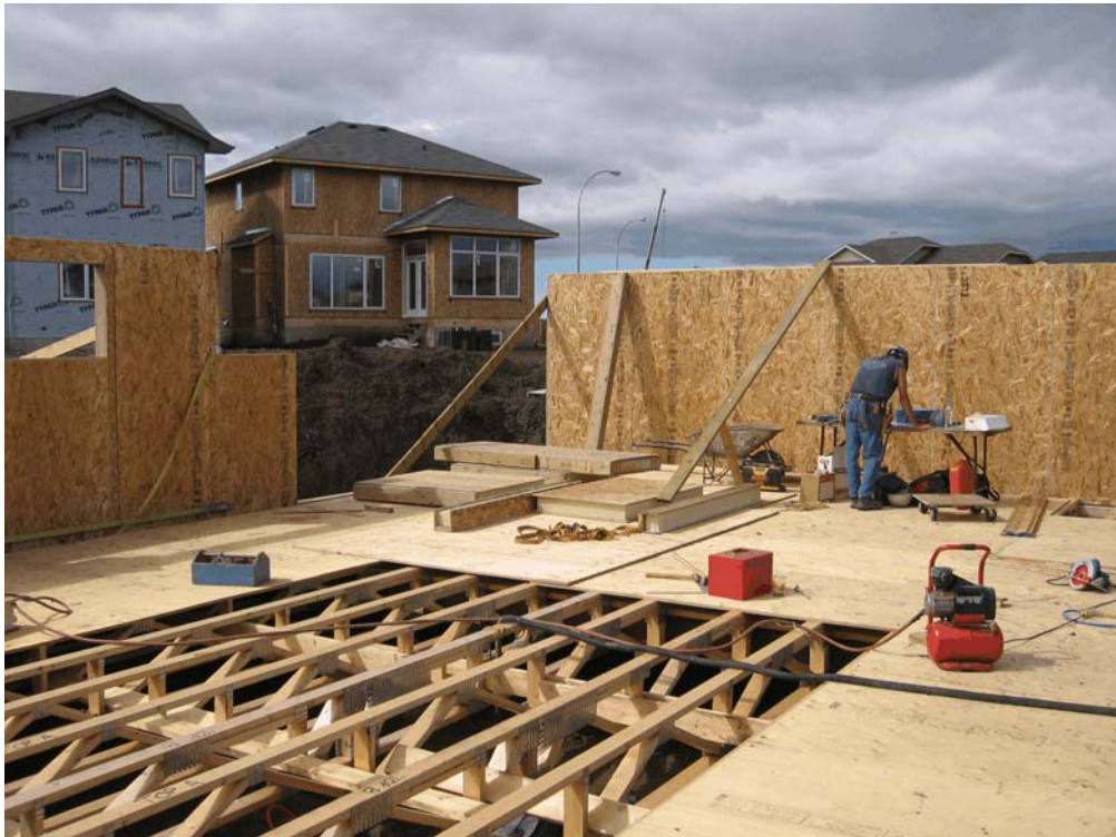
Figure 1. Factor 9 Home Under Construction—June 16, 2006 Photo Credit: Rolf Holzkaemper
