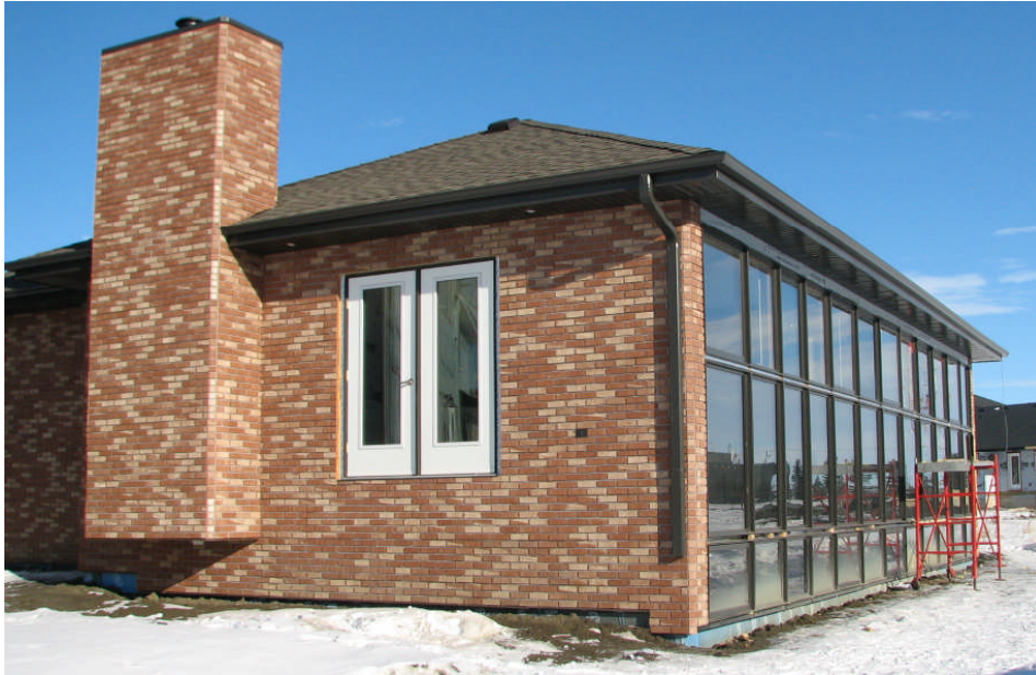
Figure 2. View from the southwest. The active solar thermal panels are in a 5 foot tall horizontal band between the upper and lower windows on the south wall of the house. Note that the eavestrough and downspout are installed. The downspout water will be piped into the flexible bladder storage tanks located beneath the basement floor. This stored water will be used for toilet flushing and exterior non-potable uses.
